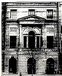
Kosciuszko Foundation House.
